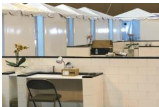
Build medical nursing stations & desks
