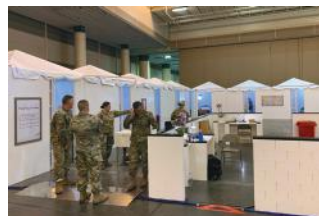
Install linear wall partitions & medical isolation pods
